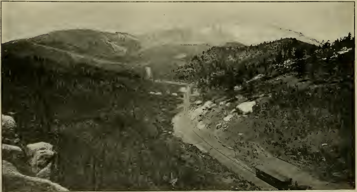
FIG. 1—VIEW OF 3\frac{1}{2} MILES OF ROADBED.
